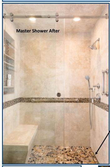
Linear drain used so the homeowners would not have to stand over the drain when showering.
